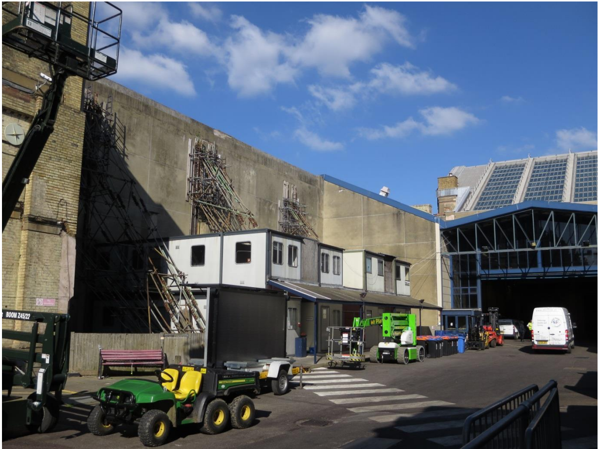
Appendix 14.2 Alexandra Palace North West Service Yard Wall Photographs
